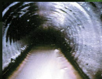
Service Water Line – Baseline Inspection
